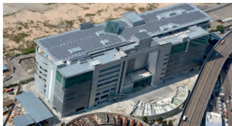
HONGKONG EMSD Headquarters
