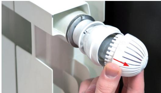
2. Use one of the limiters included in the knob cap to limit the adjustment range of the thermostatic head. By using both limiters, you can limit the the adjustment range both ways in order to lock the thermostatic head in the selected position.
