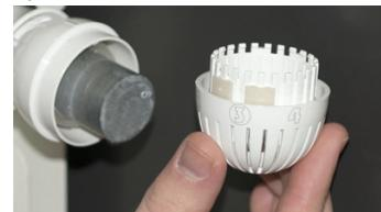
4. After the limiters have been positioned, return the knob to the initial adjustment position (**3**), applying sufficient pressure.
