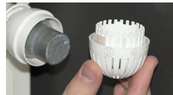
Example: Attach the limiter to the left of the number **3**. This allows the knob to be fully opened, or closed as far as **3**.
