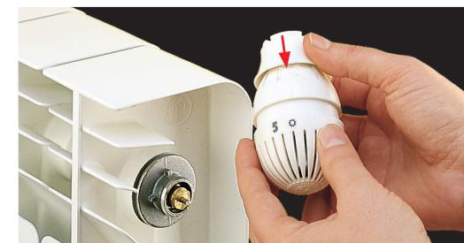
Connect the thermostatic head to the valve, making sure the valve pin (A), the thermostatic head opening (B) and the indicator line (C) are aligned.
