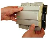
The modular design with a separate bottom plate for wiring makes the unit easy to install and commission. The bottom plate can be put into place before the electronics are installed. The controller is mounted above a false
